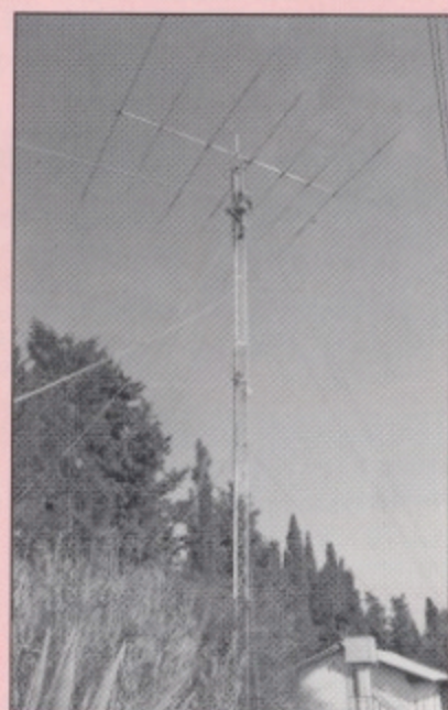
Dismounting the antenna from a height of 10m with manpower!
