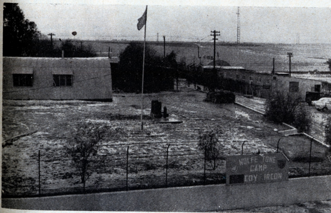
● Sixty seven windows, the roof of the signal hut and the winterization programme, were written off in the space of fifteen minutes on Friday 21 January, when a freak hailstorm hit the camp. The flowers and plants carefully
